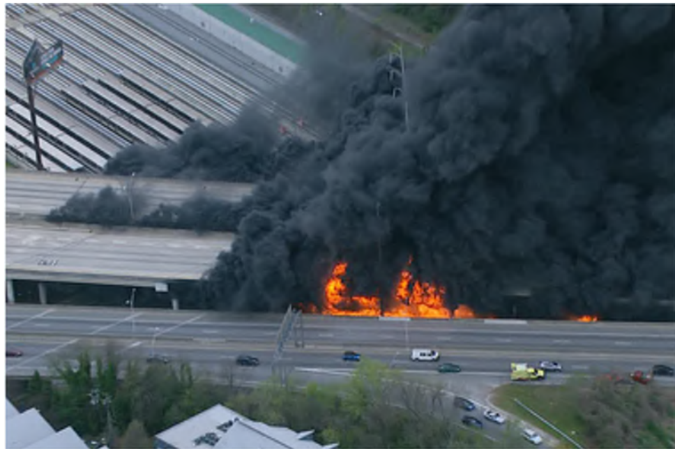
I-85 fire: Section of Atlanta highway collapses
