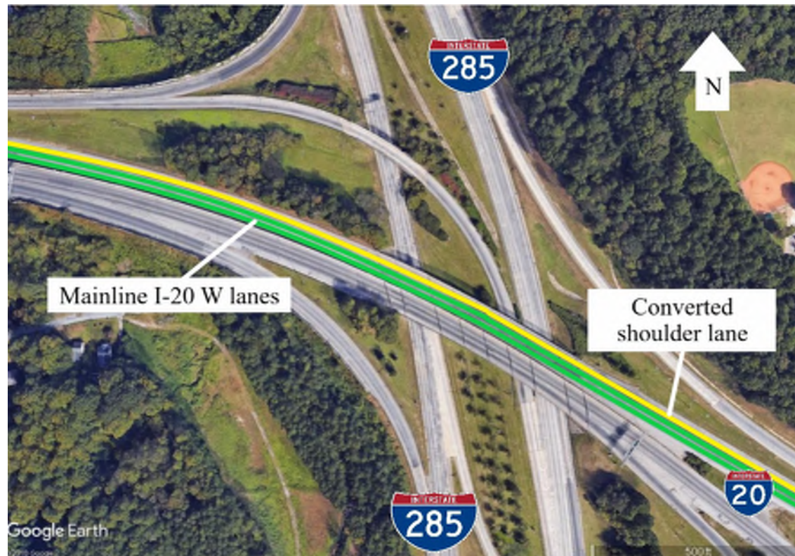
Proposed Lane Configuration of I-20 West between Exit 51B and Exit From I-285
